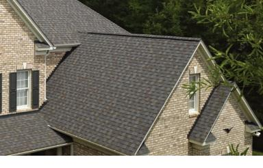
Since the early 1900s, the three-tab or strip shingle was the standard composition shingle installed on single family residences. Color was about the only appearance differentiation in this class of shingle.
